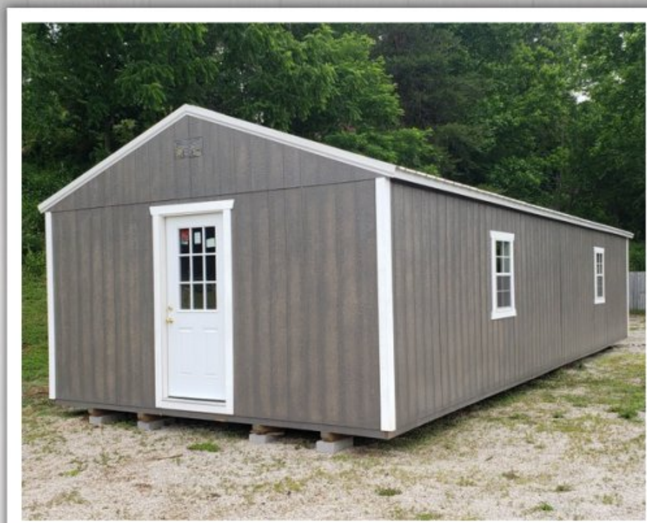
Cottage Lakeside shown in Driftwood stain.
